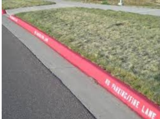
Figure 8 – Typical fire lane striping installation
