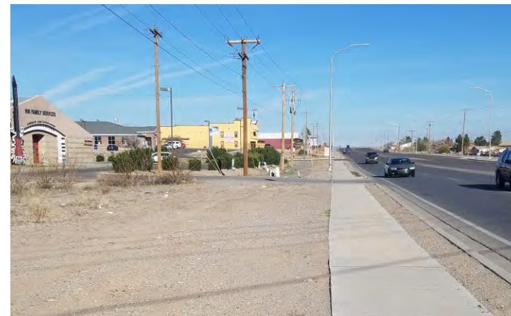
Figure 5-21 | Detached sidewalk along McNutt Rd
